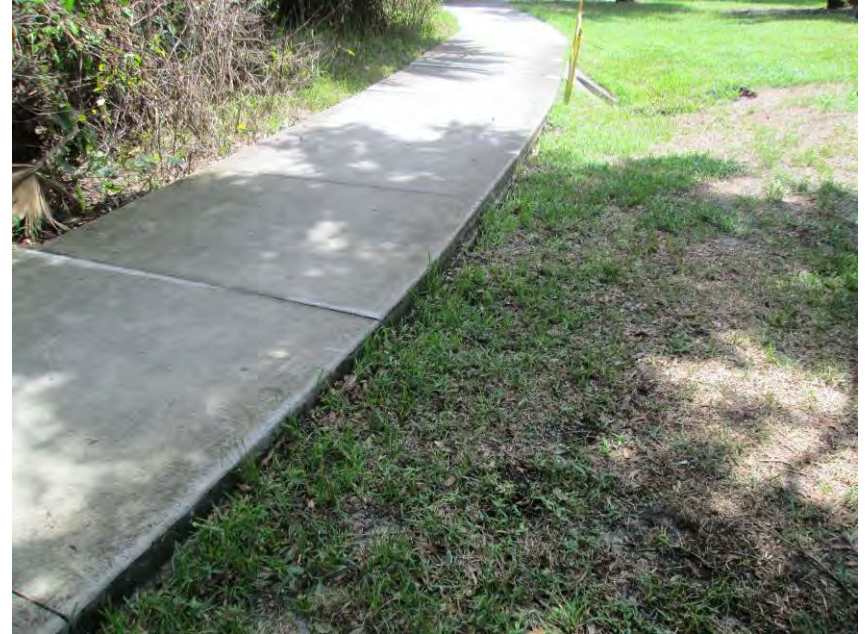
Area to backfill along nature trail
