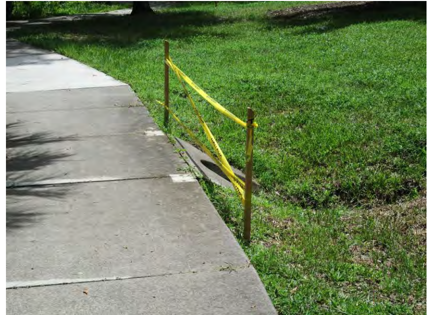
Area to install handrail
