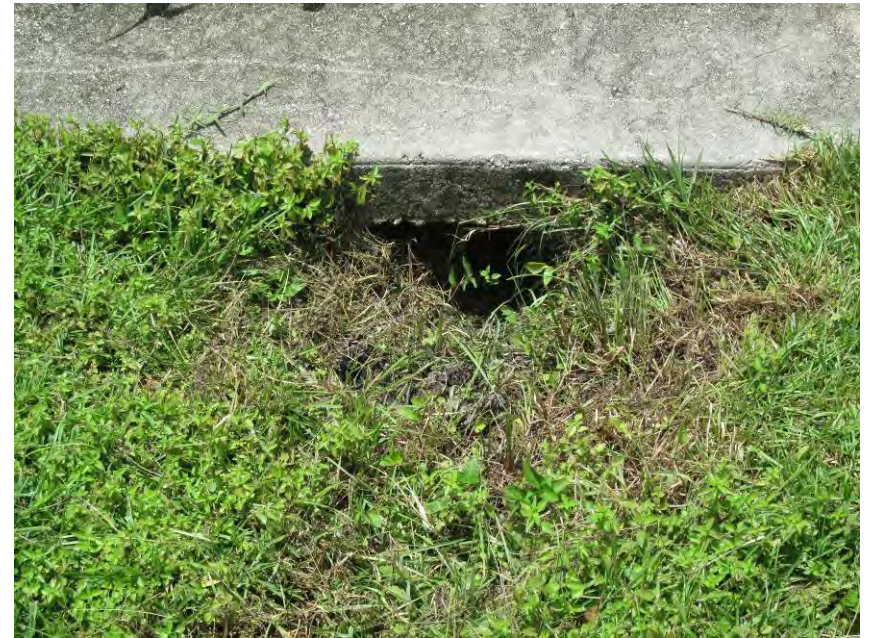
Southwest side of Mulberry Ave- clear 40'x10' of vegetation in channel, backfill & compact undermined area
