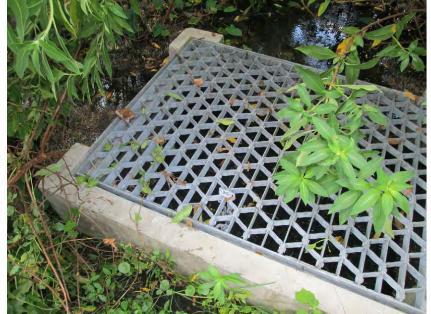
Buttercup Glen- clear 10' of vegetation on all sides of structure
