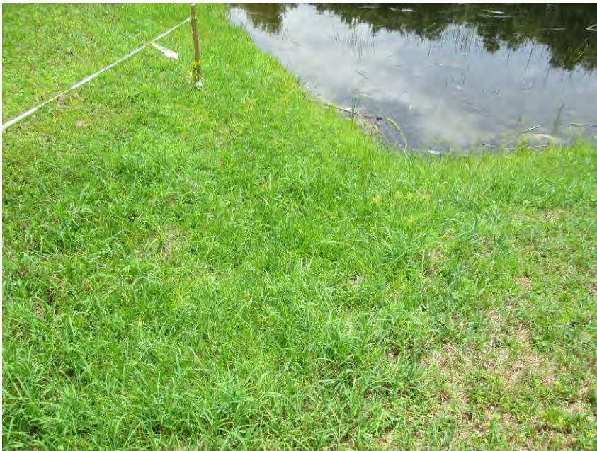
Swale erosion on northeast corner of pond 14
