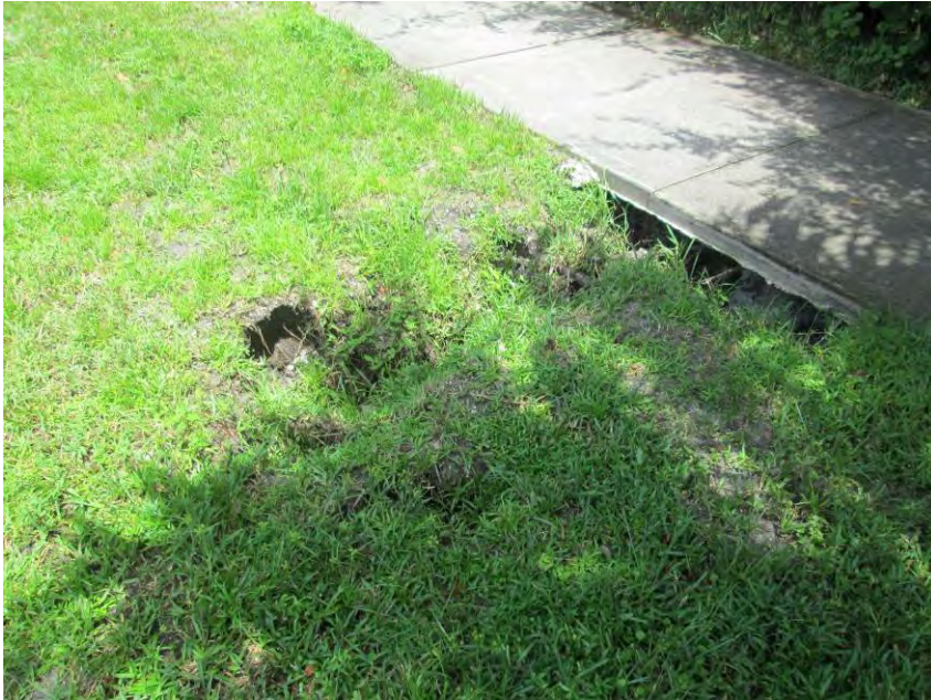
Area to install yard drain under nature trail
