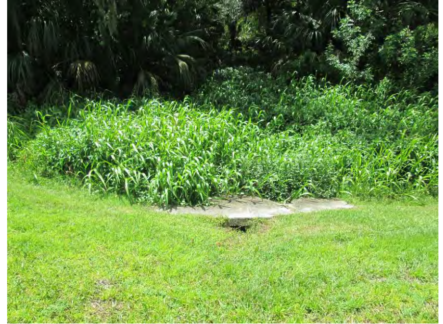
Southwest side of Mulberry Ave- clear 40'x10' of vegetation in channel, backfill & compact undermined area
